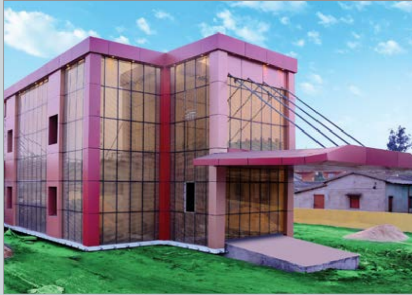
Project Name: Hotel Golden Steel City: Jajpur, Odisha Product used – Façade: SunShield Royal Gold Trendz, 5 mm thickness
