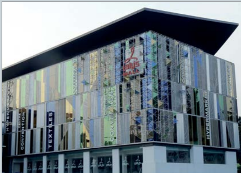
Project Name: Laly's Mall City: Pattikad, Thrissur, Kerala Products used – Façade: SunShield Royal Gold, Opal Golden Bronze, Opal Royal Blue, Opal Cool Green, 5 mm thickness Interiors: Sparkling Regal Gold, Sparkling Snow White, 6 mm thickness
