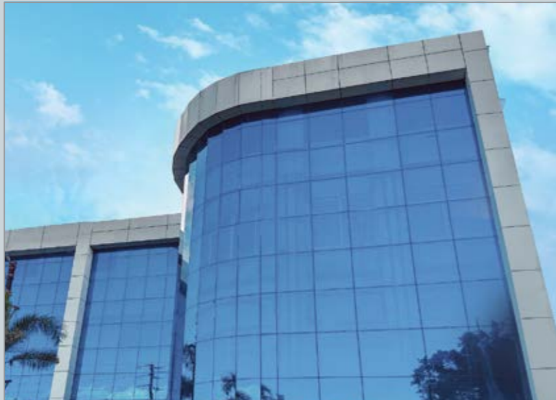
Project Name: Tamluk Library City: Kolkata, West Bengal Product used – Façade: Opal Royal Blue, 5 mm thickness
